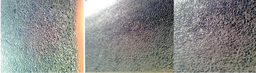
Polished aggregates At KM 1550+230 SBC
