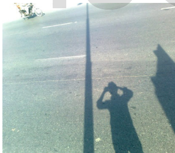
Low severity cracks At KM 1532+800 SBC
