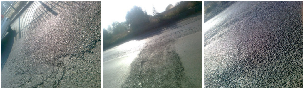
Low severity raveling At KM 1514+700 SBC
